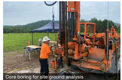
Core boring for site ground analysis
